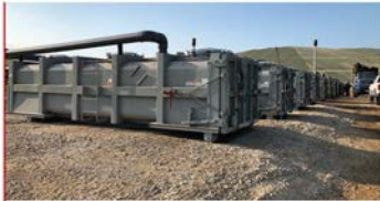
FerroSorp loaded in 10 vacuum boxes
