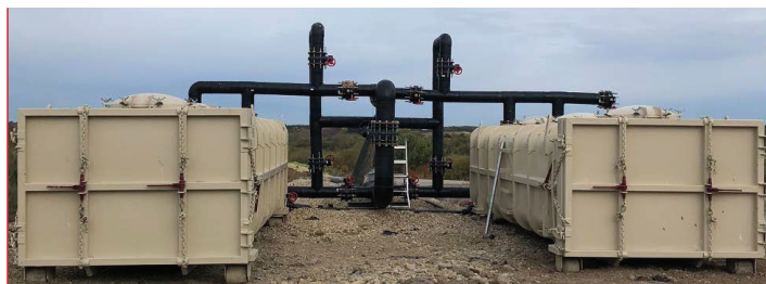
Vessels field-installed with 35,200 lbs of FerroSorp
