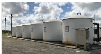
Six vessel H 2 S removal iron sponge system
