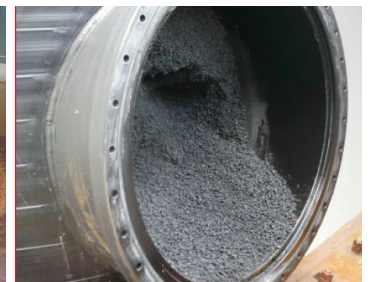
Spent FerroSorp can be vacuumed out of vessel
